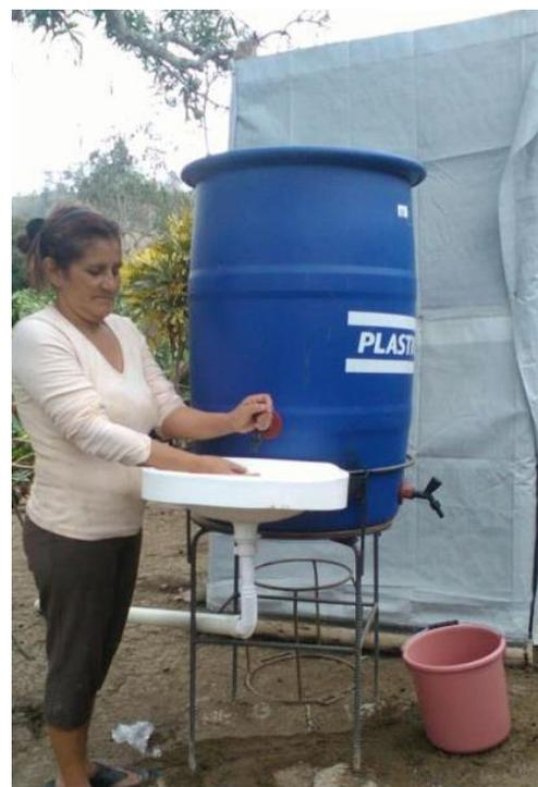
*Photo 2: Handwashing facilities connected to water tanks*
